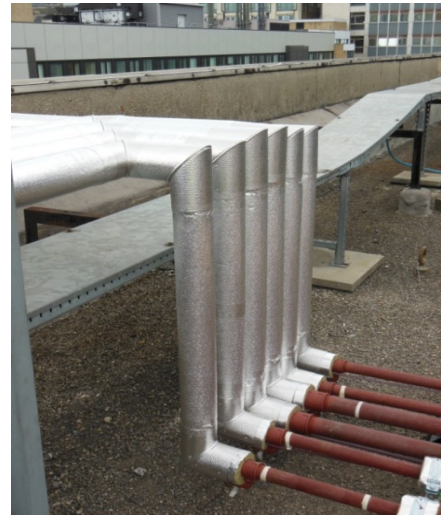
Figure 16.1 Typical external pipework details with Venture Clad finish and Hammer-Clad bend covers fixed with self-tapping screws
